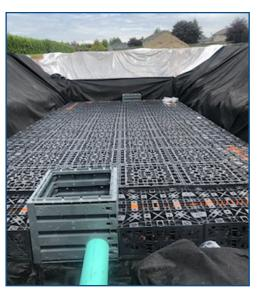
The base layer consists of both Ecobloc light & flex, with two Vario shafts also installed for inspection and cleanout access. Each block is stacked along the base layer, secured with connector elements and end plates. An extension was added to the Vario shaft and the final layer was added. The site was then evenly backfilled with gravel as per manufacturer guidelines.
